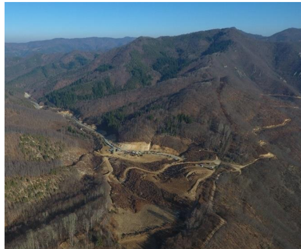
Border Crossing Check Point Dimario - Rudozem panoramic view of on-going works
